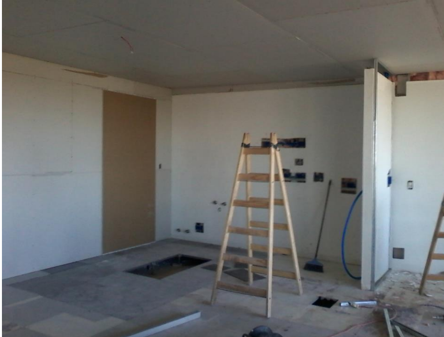
Coffee area: secondary entrance closed, connection with existing pantry and gypsum boards placed in ceiling
