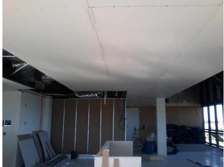
Gypsum board ceiling placed
