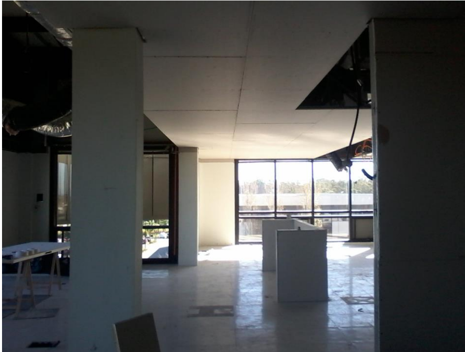
Gypsum board ceiling placed
