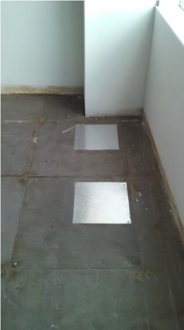
Open Office: Technical floor repaired.-
