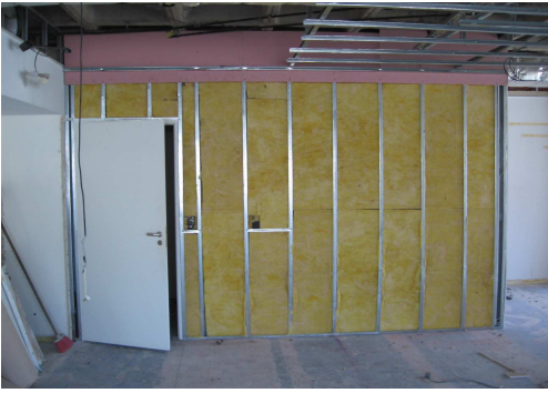
DATA CENTER FROM OUTSIDE - DRY WALLS - METAL STRUCTURE - GLASS WOOL FOR THERMAL AND ACOUSTIC INSULATION - RED GYPSUM BOARDS (FIRE RESISTANT)
