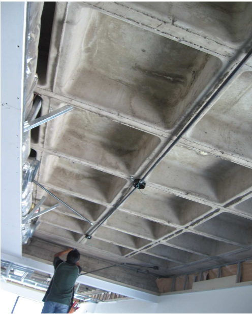
OPEN SPACE - NEW ELECTRICITY PIPES (STEEL)
