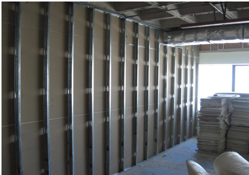
TRAINING ROOM FROM INSIDE - DRY WALLS - METAL STRUCTURE + DOUBLE GYPSUM BOARD
