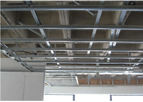
KITCHENETTE - CEILINGS - METAL STRUCTURE
