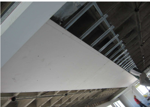
OPEN SPACE - CEILINGS - METAL SRUCTURE + GYPSUM BOARDS
