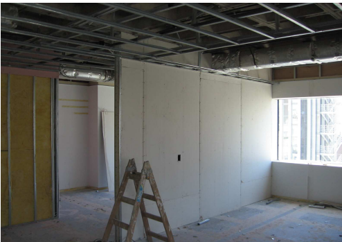
MANAGER'S OFFICES - DRY WALLS - METAL STRUCTURE + GYPSUM BOARDS
