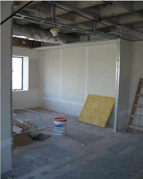
MEETING ROOM FROM OUTSIDE - DRY WALLS - DOUBLE GYPSUM BOARD FOR ACOUSTIC INSULATION
