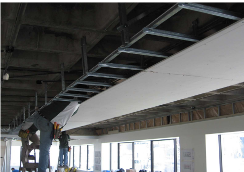
OPEN SPACE - CEILINGS - METAL SRUCTURE + GYPSUM BOARDS
