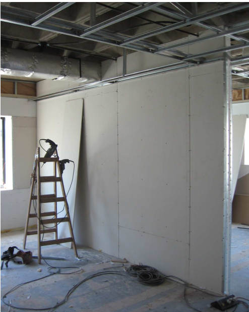
MANAGER'S OFFICES - DRY WALLS - METAL STRUCTURE + GYPSUM BOARD
